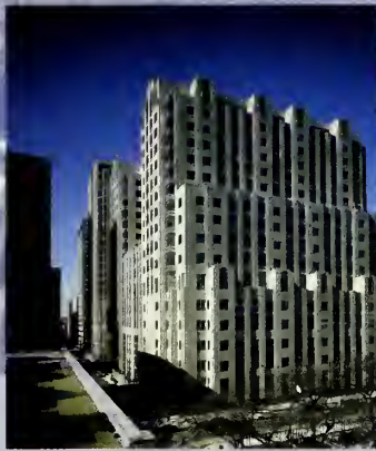
NORTHWESTERN MEMORIAL HOSPITAL CHICAGO, ILLINOIS
